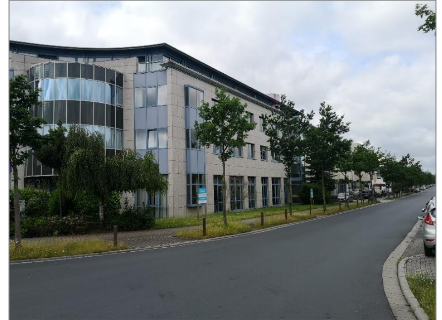
R&D Office, Germany
