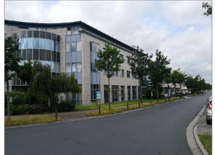
R&D Office, Germany
