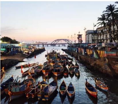
Infrastructure and illumination work at Cleveland Jetty, Worli Koliwada, Mumbai
