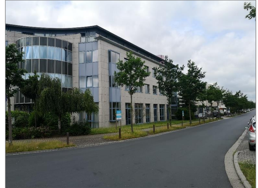
R&D Office, Germany
