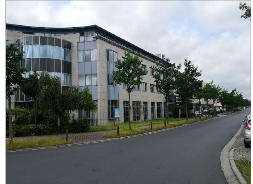
R&D Office, Germany
