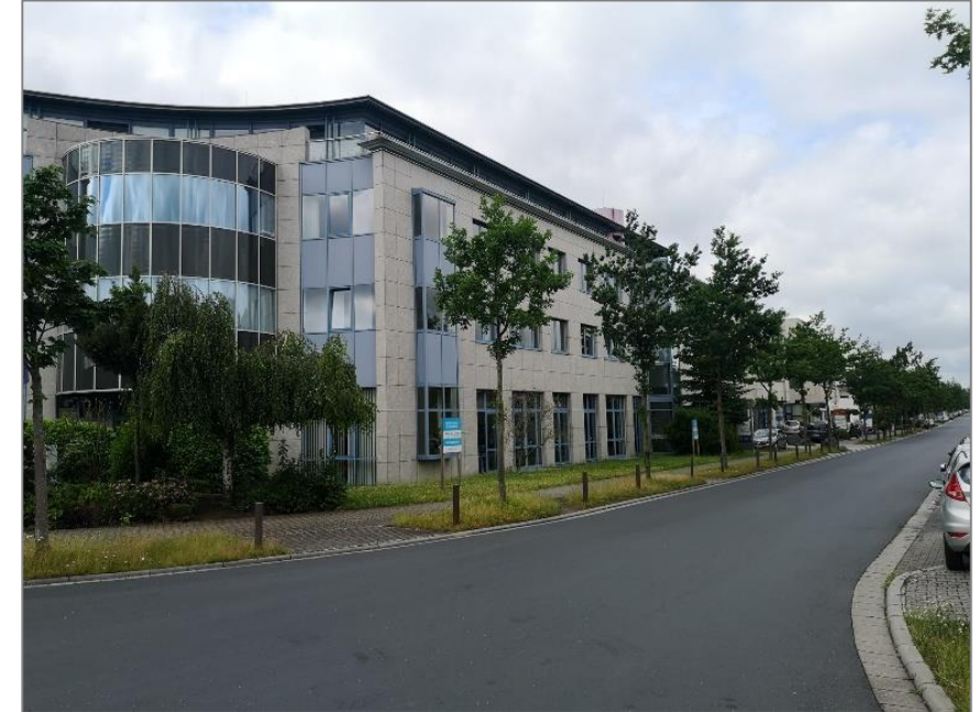
R&D Office, Germany
